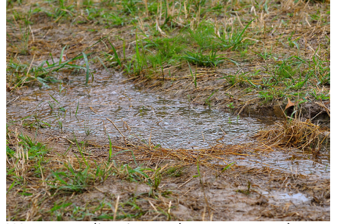
Water pooling in yard; recommend drainage
